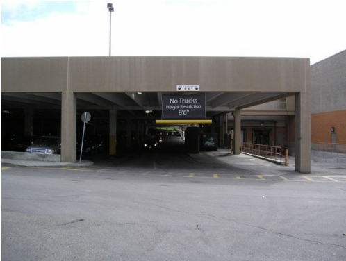
(a) Tunnel Environment
